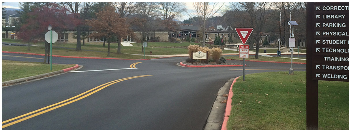
Multiple lanes of traffic merging at single intersection creates confusion with correct direction of travel.
