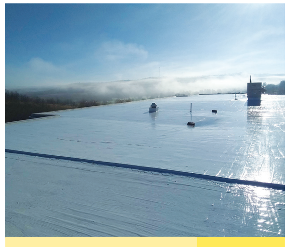
BCC Roof Renovations
